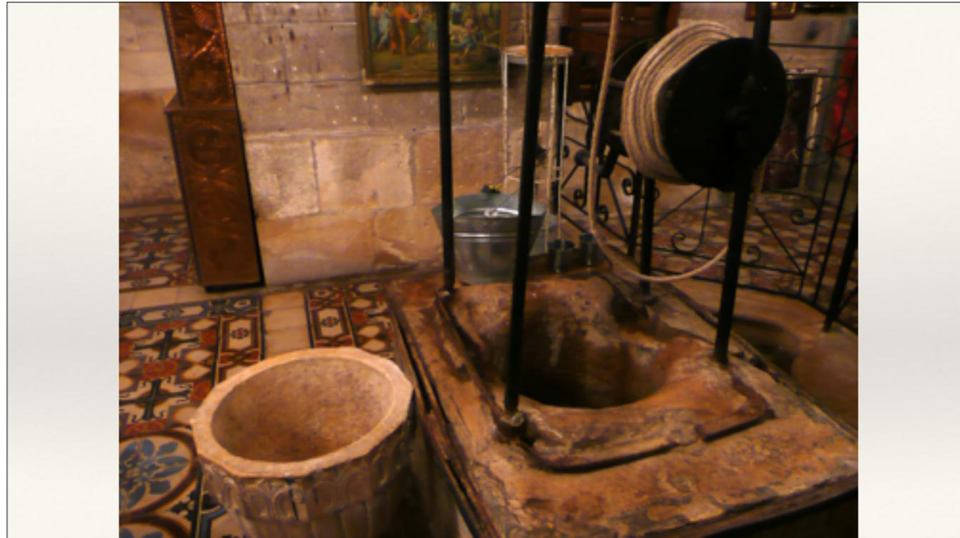
A well is still there today. It is enclosed in a Greek Orthodox church. It is a deep well at 135 feet. It is dug through the soil and into limestone rock at the bottom. The water is about 15 feet deep which means that there is 120 feet from the top of the well to the water. The area also has a number of springs and there was even a spring in the village of Sychar. Why dig a deep well there? Maybe the quality of the water was significantly different.
